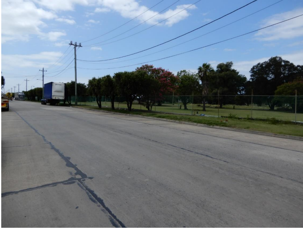
Photograph 1: Illustrating the location and context of the trees along Devon Street.
